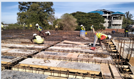
Construction Site of New Cath Lab in Eldoret, Kenya
